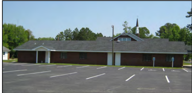
Rear elevation of the Fellowship Hall
