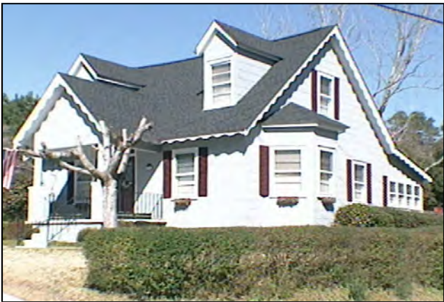
2002 Brunswick County Tax Office photo showing east elevation with bay window, enclosed rear porch, and trimmed hedgerows
